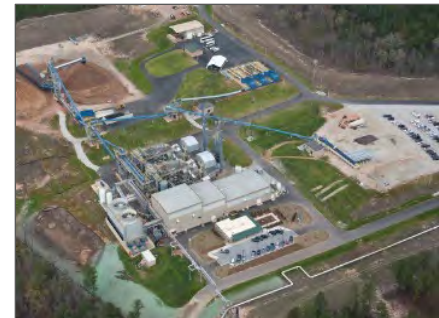
Under a $795 million ESPC – the largest renewable-energy ESPC in U.S. history – Ameresco replaced coal-fired cogeneration facilities at the U.S. DOE's Savannah River
