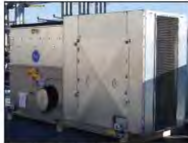
Intake and Discharge Sound Attenuation
