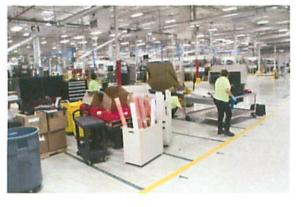
The repairable contents were kept in storage pods to remain onsite. Bobcats were used to move the unsalveageable contents. All storage and locker systems that could be saved were also relocated to a staging area for cleaning. Commercial negative air units and commercial dehumidifiers were used to remove the moisture and dry out the contents and structure.
