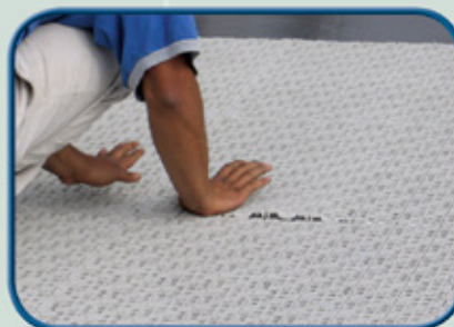
Install PDS tiles
