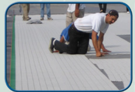
Install PDS tiles across center of field
