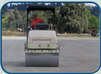
Laser grade and compact to 95% proctor
