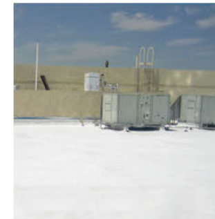
Pyramic® Plus Lo reflective coating reduces your buildings heat gain.
