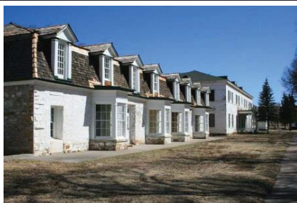
Fort Stanton Stabilization
