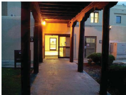
VA Hospital Historic Walkway Restoration
