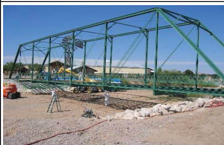
Rio Hondo Bridge Relocation
