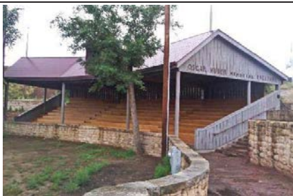
Madrid Grandstand Rehabilitation
