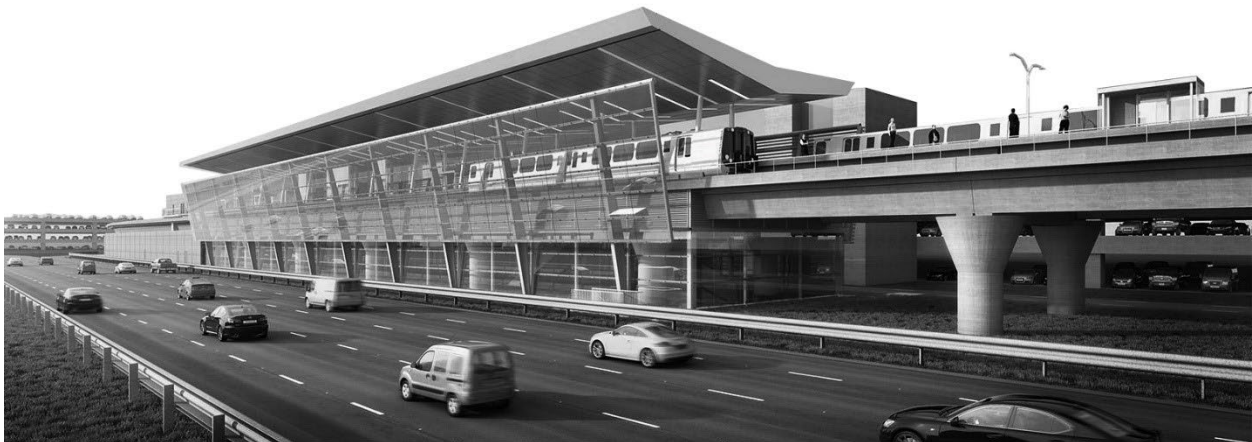
Figure 4. Dulles Corridor Metrorail Silver Line Extension, Phase 2. Throughout Phase I and now into Phase II, IBTS continues to support the Virginia Department of General Services and Metropolitan Washington Airports Authority with thousands of code compliance inspections, making mass transit a viable alternative for hundreds of thousands of residents in the DC Metro area.
