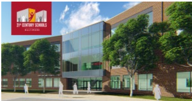
Figure 3: Patterson High School & Claremont Middle/High School, Baltimore (new construction). IBTS is providing all code compliance reviews and building code inspections for 28 Baltimore City public schools totaling 3 million square feet.
