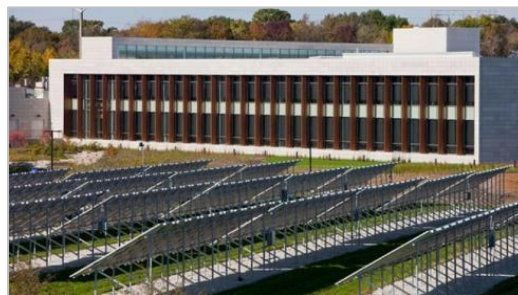
Johnson Controls headquarters in Glendale, Wisconsin
