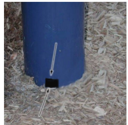
Playground manufacturers supply marks or stickers on uprights to indicate adequate surfacing levels.
