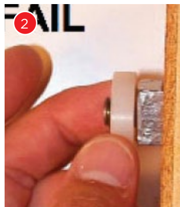
This bolt end is an unsafe protrusion.
