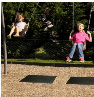
Wear Mats under swings can help keep loose-fill materials in place and protect unitary surfaces from wear.
