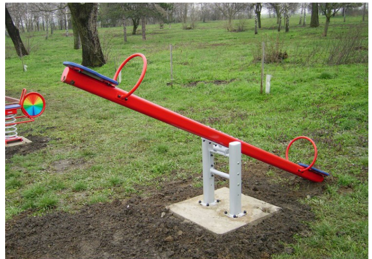
In addition to having unacceptable surfacing around it, this seesaw's exposed concrete footing and potential pinch point poses a hazard to children.
