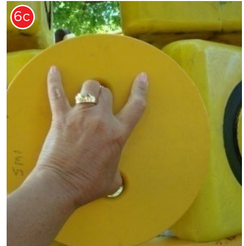
The head probe does not freely enter; therefore, this tic-tac-toe panel poses a head entrapment hazard and should be corrected.
