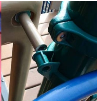
Hardware is missing and causing the component to come apart.
