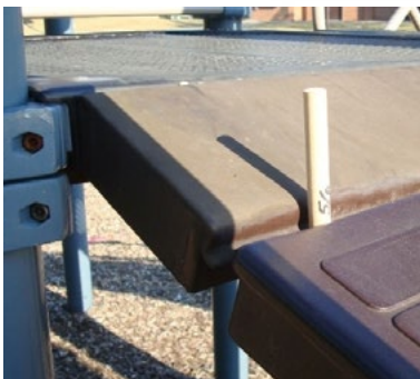
Demonstration of test for crush and shear hazard.
