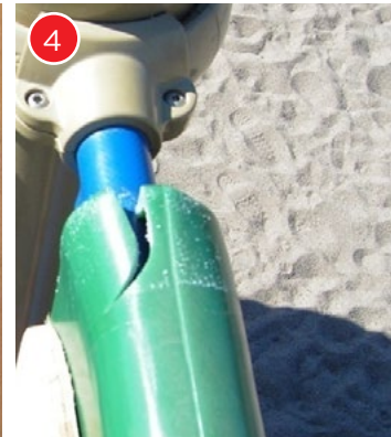
This cracked component is a hazard.
