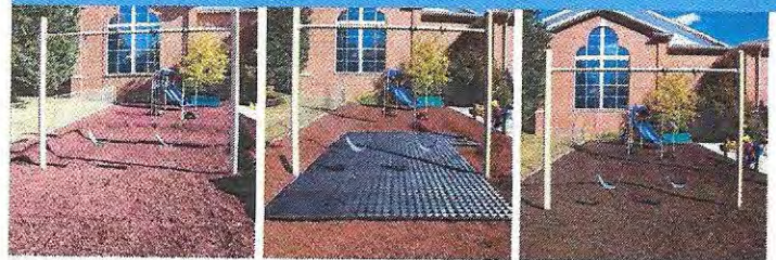
3" of mulch placed
