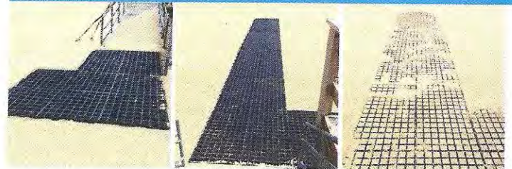
excavate 3" of sand
