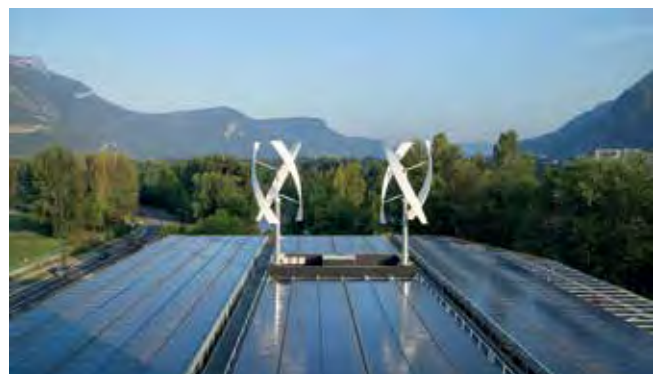
Solar and wind-powered roof at IntenCity facility in Grenoble, France
