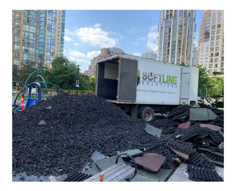
Softline Solutions Re-Cycle Generation Two process includes removal of existing surface and recycling the product onsite for use in a new surface.
