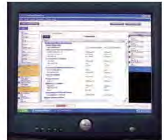
Factory-testing ensures that all controls work appropriately.
