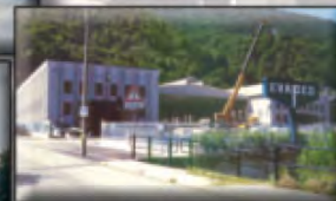
EVAPCO Europe S.R.L. Sondrio, Italy
