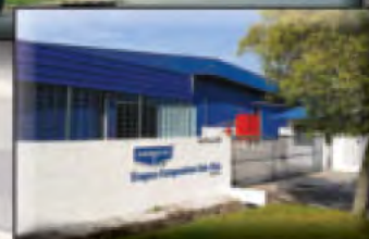
EVAPCO Pacific Selangor, Malaysia
