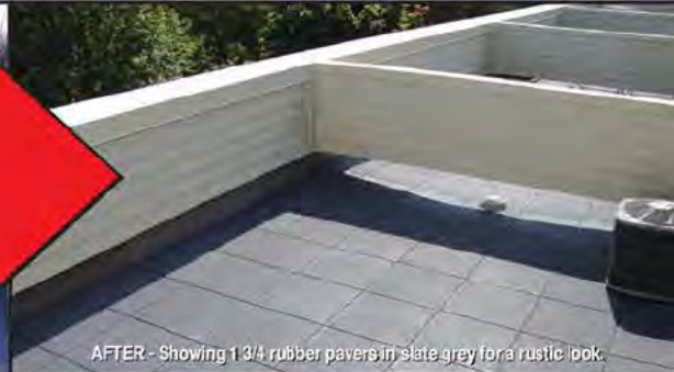
AFTER - Showing 1 3/4 rubber pavers in slate grey for a rustic look.
