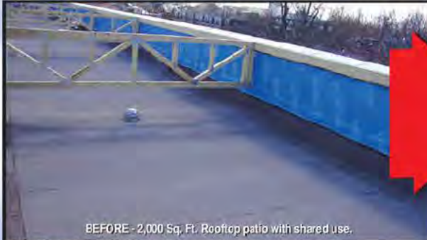
BEFORE - 2,000 Sq. Ft. Rooftop patio with shared use.
