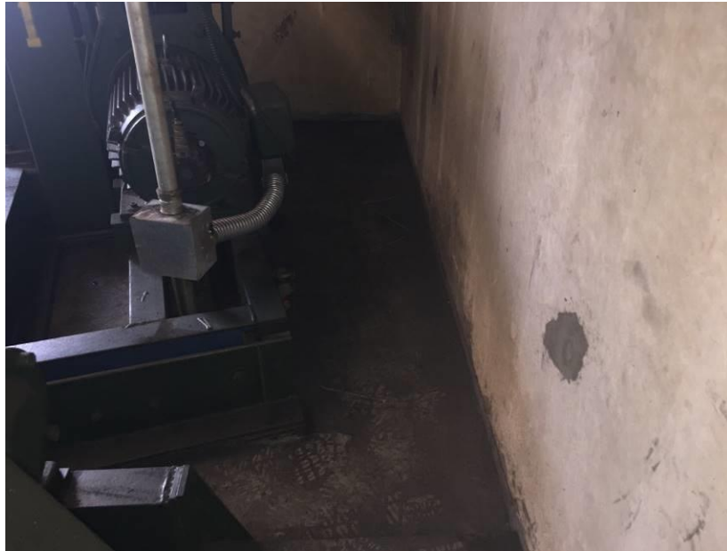
Dirty Machine Room
